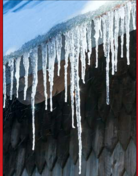
RX Roof & Gutter De-Icing
