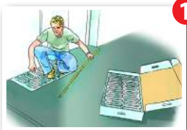
Lay out Reflect Plates
