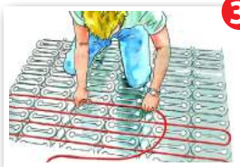
Install heating cable in grooves, pressing gently
